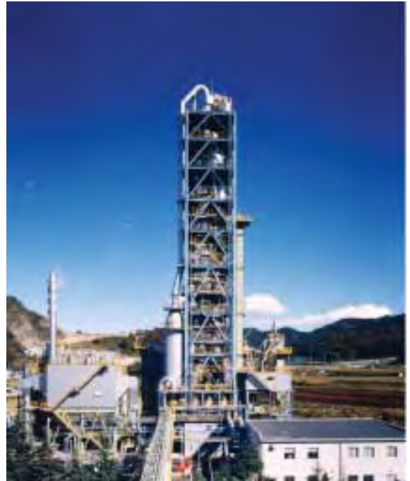
Photo 2 Overview of 200 t/day plant
